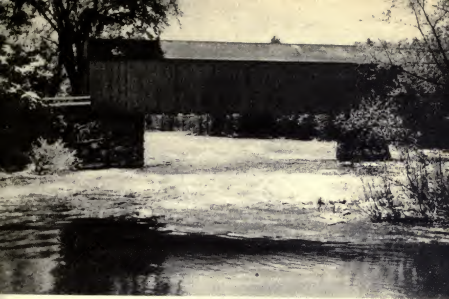
HART'S BRIDGE, WEST CORNWALL
